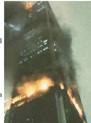
The Interstate Bank Building fire consumed several floors but did not damage the steel superstructure.
